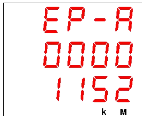
Fig.3.2.12 Setting the base value of total phase A active energy
